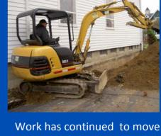
Work has continued to move forward on the repairs to the West end of the basement. Crews from Lowe Excavating came and unearthed the foundation on the east and north walls of the building, tore out the "dog house" entry, and made all of the repairs needed in that area and then back filled the space.
